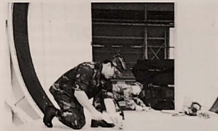
(Foreground) TSgt. Darren Kennedy, structural craftsman for the 507th CES, works with a Guardsman constructing a stage in one of the areas for activities.
